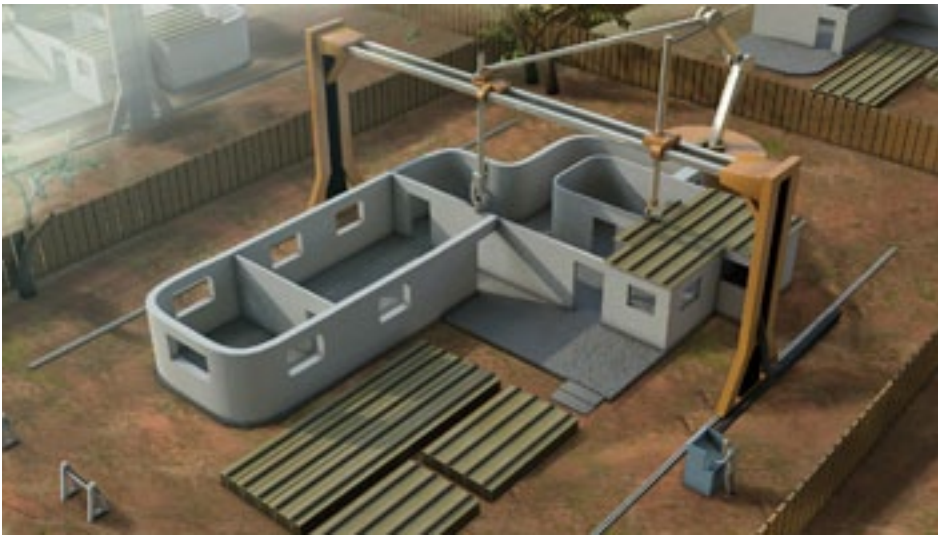
Example of contour crafting. Note for scale the figurine of the human operator at the console at bottom right.
