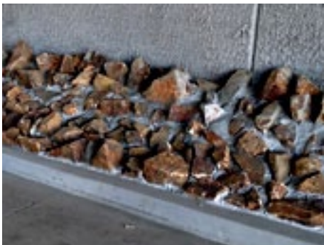
The rocks installed on the margins of the I-5 underpass. From the Facebook page of Homelessness News San Diego
